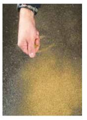
**ARDEX Aggregates** are for use with ARDEX Subfloor Smoothing compounds where thicker applications are required, or for fully blinding epoxy primers.
