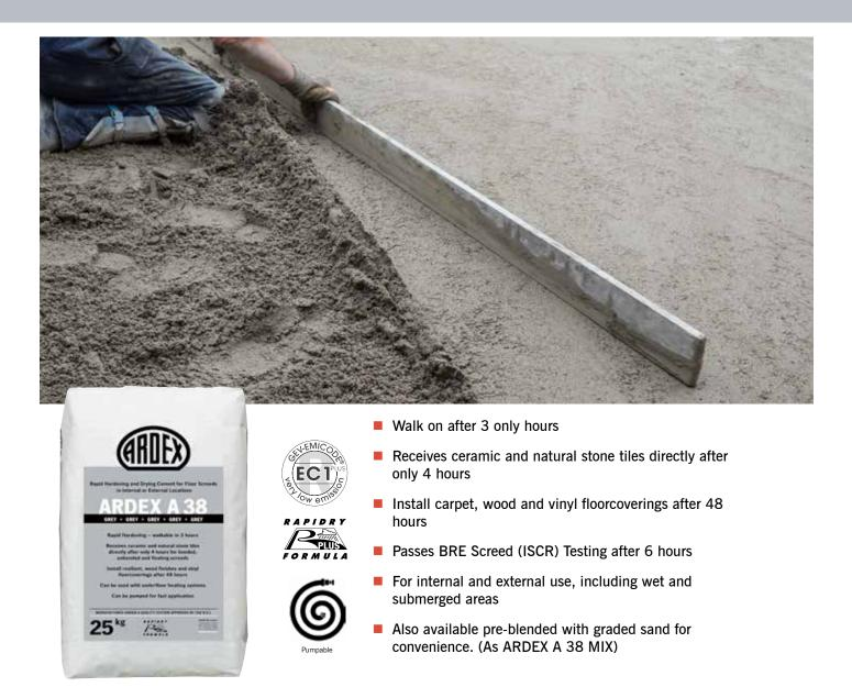
**ARDEX A 38** produces ultra-rapid drying floor screeds which can be walked on after just 3 hours and floorcoverings installed in as little as 4 hours, regardless of thickness.
