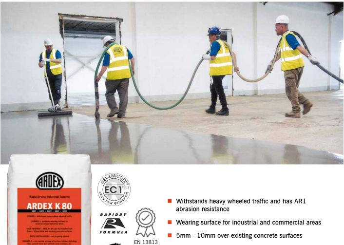
Can receive a range of surface finishes including suitable resin coatings, tiles and natural stone and paint
