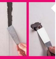
Reinforce joints that tend to crack with the ARDEX self adhesive mesh scrim. Apply the mixed ARDEX WPC (MIX No.1) with a spatula, pallet knife or trowel to seal joints in corners and fill holes and gaps around pipes, and leave to harden for approx. 1 hour prior to applying the first coat of Mix No.2.
