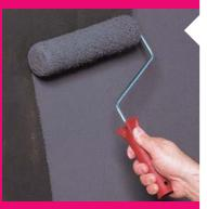
Mix approximately 0.75kg ARDEX WPC liquid with 0.75kg ARDEX WPC powder for every m² at 0.8mm thickness to obtain a flowing consistency. Apply this Mix No.2 evenly with a brush or paint roller to cover the surface with a uniform coat. A second coat should be applied approximately 30 minutes after the first coat to obtain an effective waterproof protection layer of at least 0.8mm thickness. ARDEX WPC will dry to a dark brown flexible coating.
