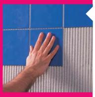
Ceramic tiles can be fixed onto the second coat of ARDEX WPC after approximately 60 minutes.
