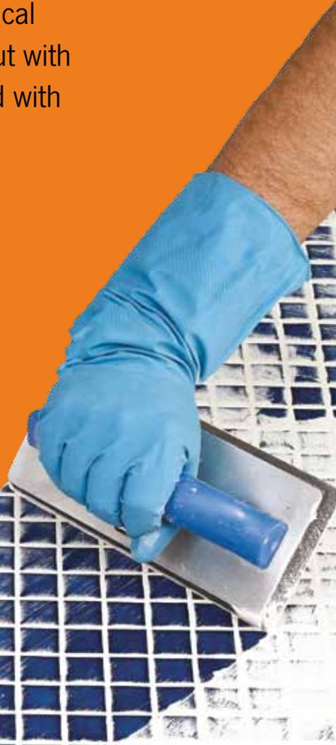
**ARDEX EG 8 is a cement/epoxy hybrid grout and adhesive with excellent resistance to most chemicals but, unlike traditional epoxy grouts, ARDEX EG 8 is easy to apply, requires no special tools, and can be cleaned off the tile surface up to 45 minutes after application.**
